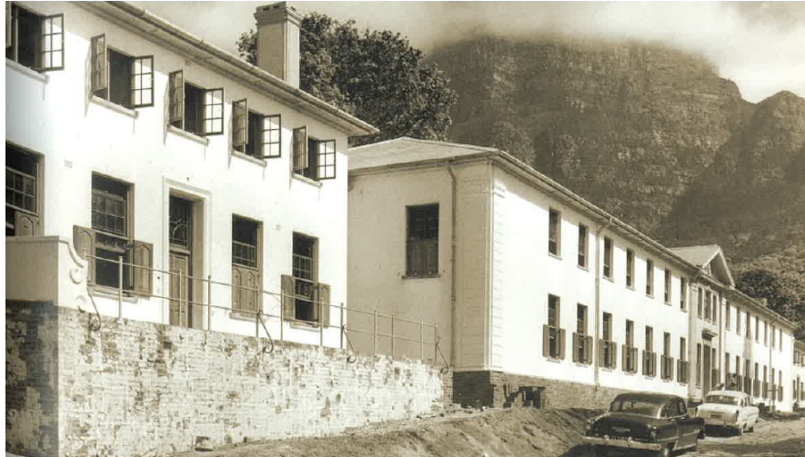
The third Rosedale, in Newlands, in the final stages of construction in the late 1950s
